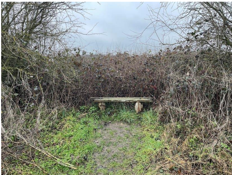
Image of a rotten bench requiring replacement.
