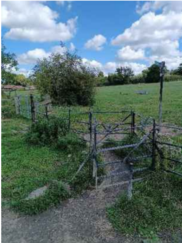
Image 15: estate fencing gate in centre of site.
