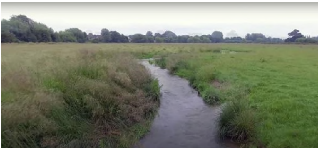
Figure 1. Example of a bypass channel designed to replicate a natural channel, River Great Ouse, Stony Stratford, Buckinghamshire (photo – Five Rivers).
