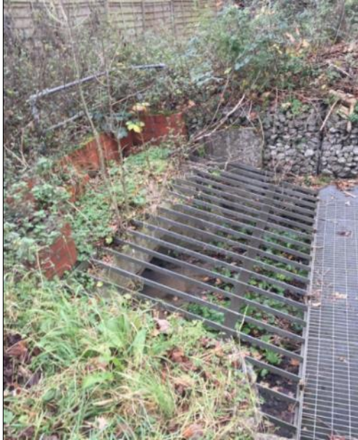
Trash screen on Bushy Mill Lane
