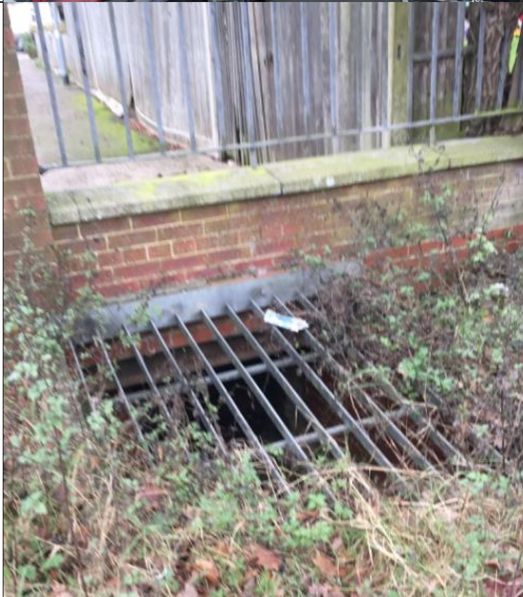
Culvert along Haydon Road at the entrance to Attenborough Fields
