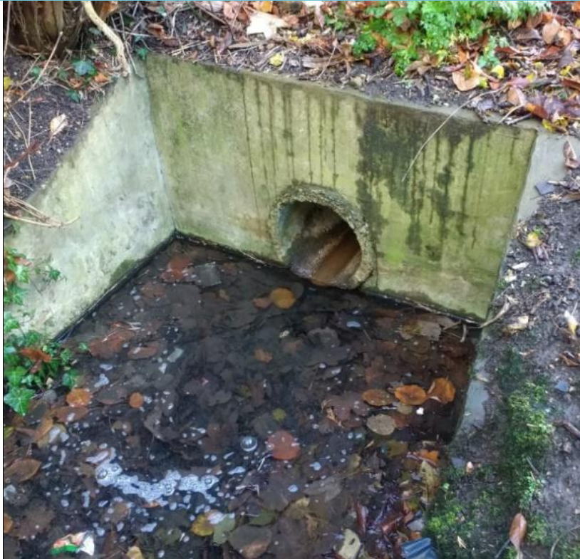
Bragbury End culvert outlet
