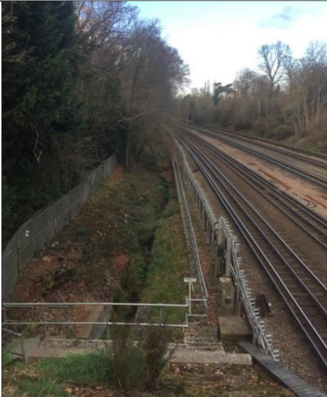
Railway and culvert exit alongside track
