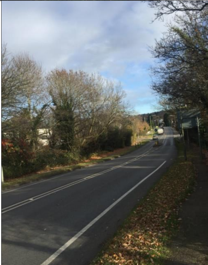
Slope down St Mary's Avenue
