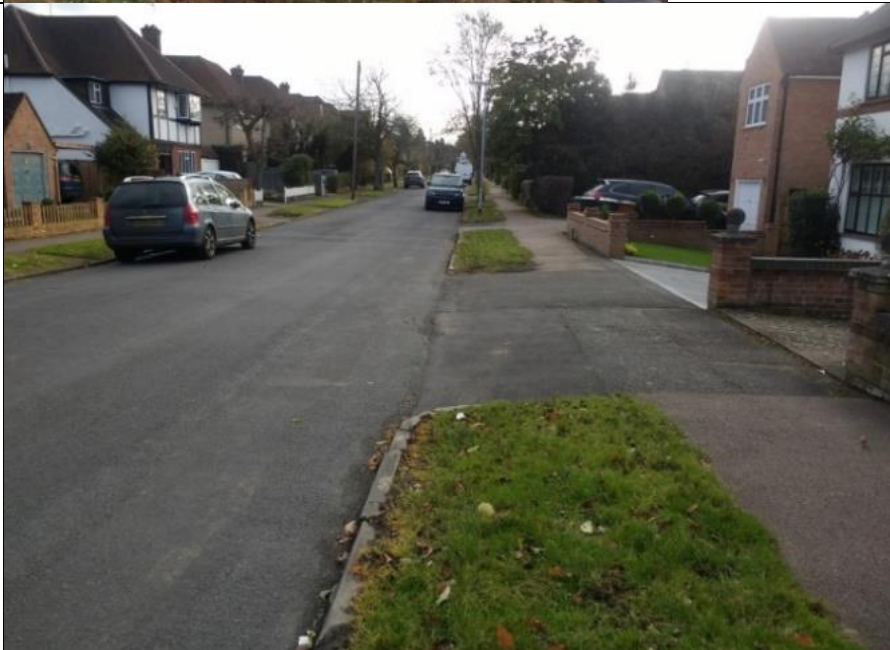
Reported flood events have occurred along St Mary's Avenue
