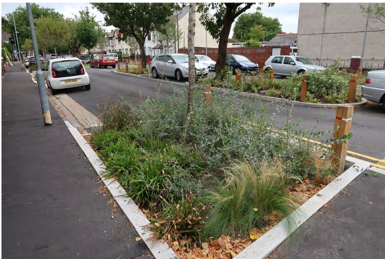
Figure 5-7: Example of rain gardens in a residential street (CIRIA, 2018 5 )
