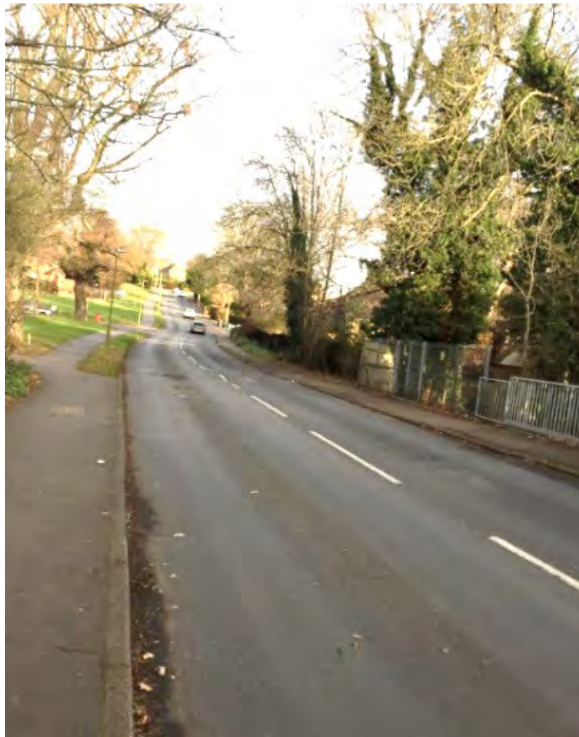
Figure 5-18: Slope in road along Raglan Gardens
